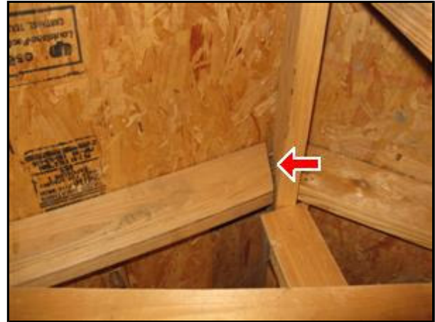
D. Picture 6 Right rear of home
