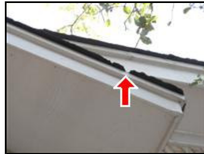
C. Picture 4 Lower left roof corner
