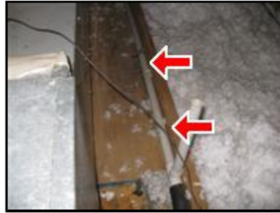
B. Picture 2 A/C condensation line
